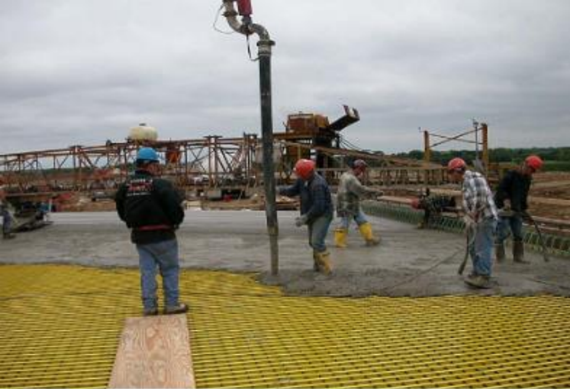
Fig. 13. Pouring and vibration of concrete at FRP reinforced bridge deck.
