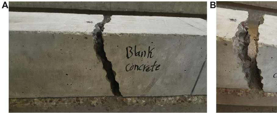
Fig. 8. (A, B): typical fracture of unreinforced concrete.
